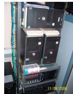
top: phone system equipment in Shawnee County; bottom: backup power supply (left), units of the computer-aided dispatch system (top), and the recorder system (bottom) in Coffey County
