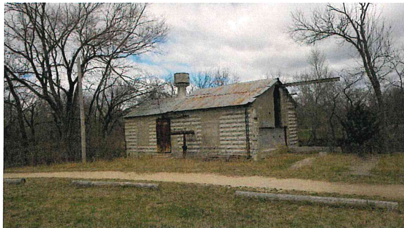
Water distribution building
